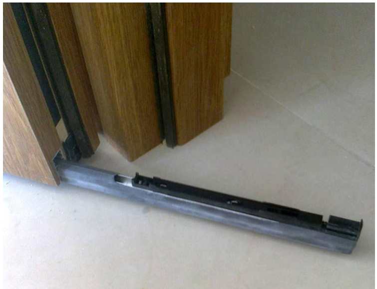
Soundproof door with retracted drop-seal
